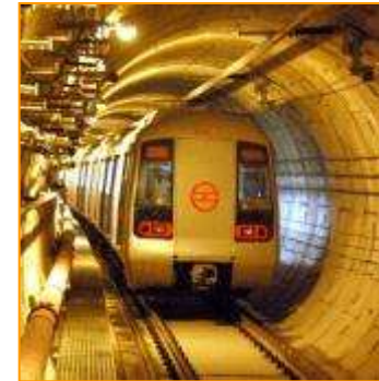
Delhi Mass Rapid Transport System Project (India)
